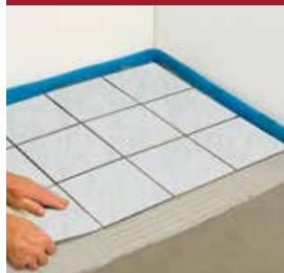
INSTALLING THE NATURAL STONE
