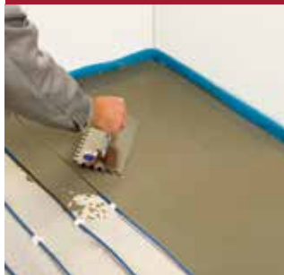
APPLYING LEVELLING COMPOUND
