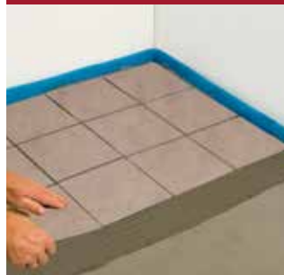
INSTALLATION OF TILES
