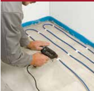
INSTALLING OF THE HEATING CABLE
