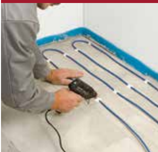
INSTALLING OF THE HEATING CABLE
