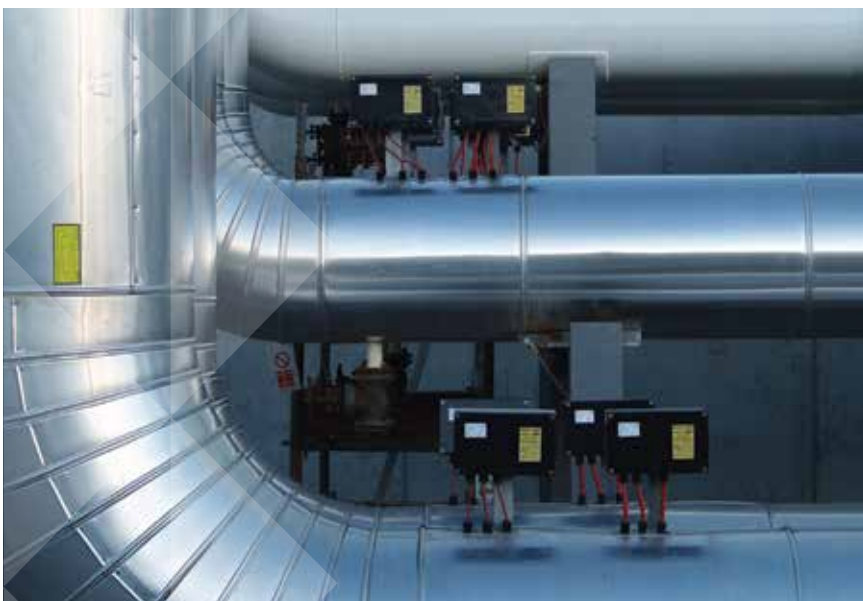
Complete and fully certified heat-tracing solution with easy-to-install connection system for long transfer lines.
